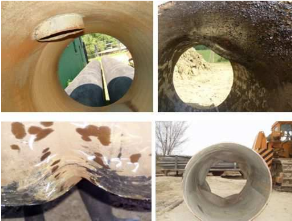
Figure 5 – Results of gas mains inspection with geometric pistons
