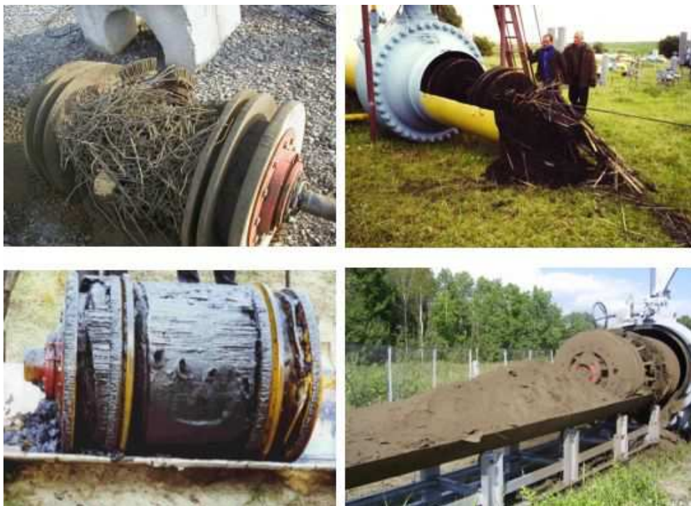
Figure 3 – Results of gas mains cleaning
