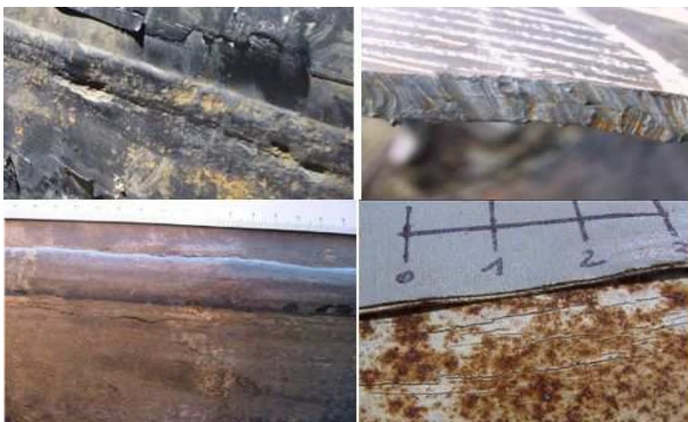
Figure 8 – Defects of a pipe body revealed with AFD pistons
