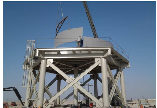
Figure 2 – General view of storage constructing process made in Saudi Arabia
